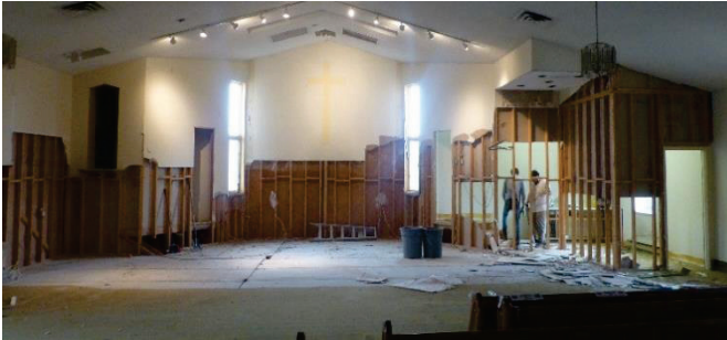
Demolition of upper sacristy and removal of inner walls
